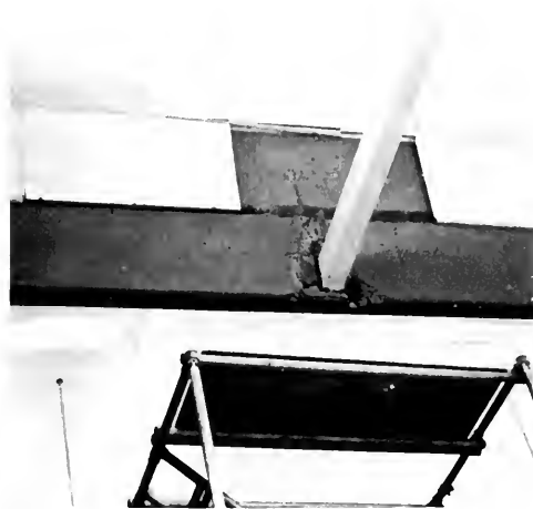
Photo 15. Sylmar High School Gymnasium. Damage to prestressed concrete beam at gymnastic equipment cross beam.
